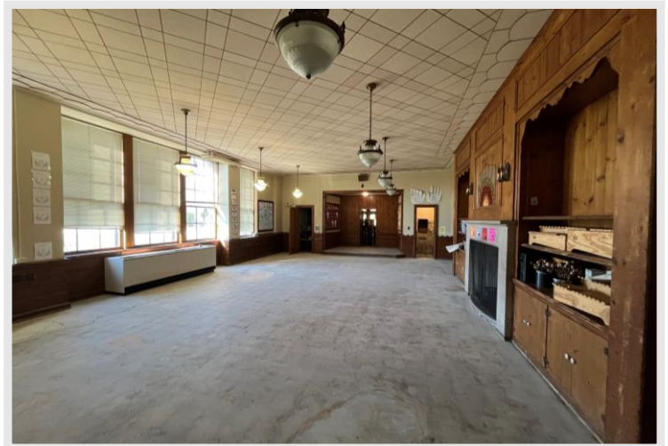
Environmental work and flooring removal in the Music Room is complete!
